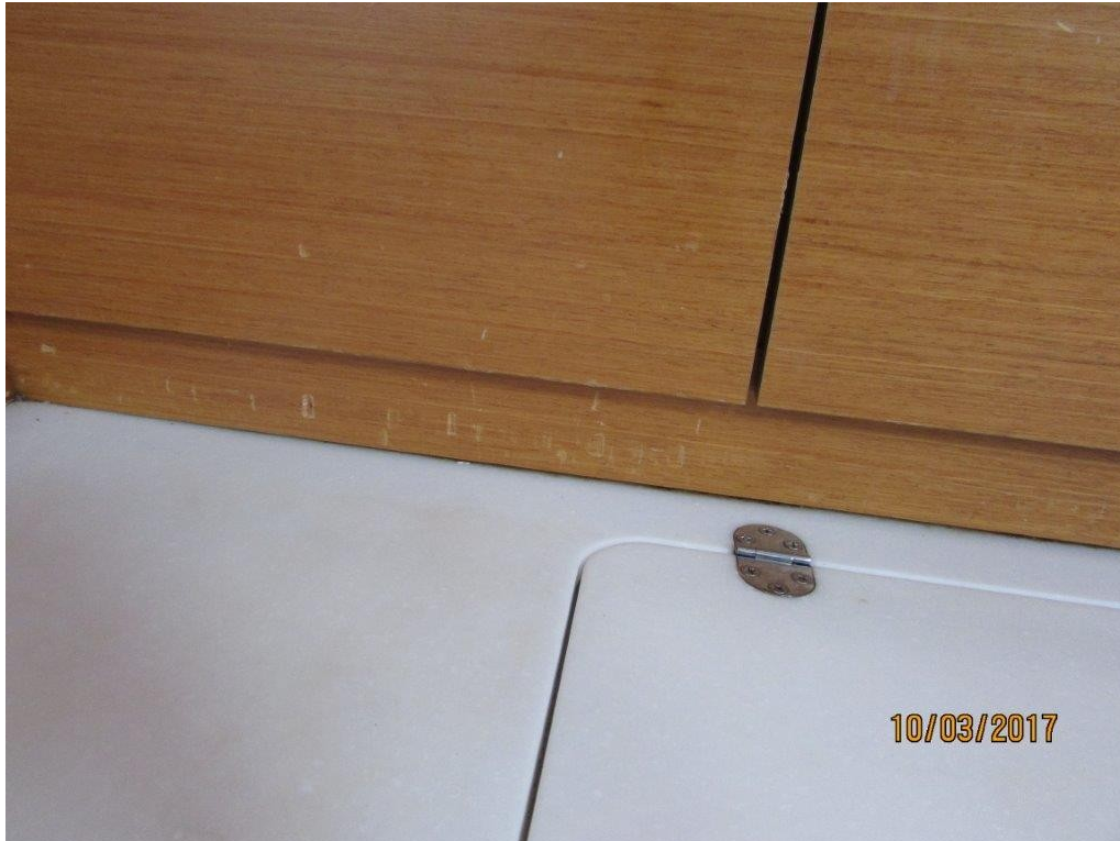
Damage to the galley woodwork not reported.
